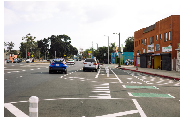
New street configuration on Broadway south of Manchester
