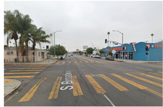
New signal installed at Broadway/67th St
